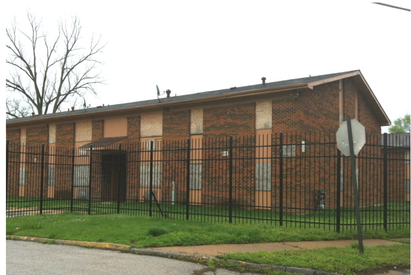
Boaz Apartments was recently foreclosed upon and is currently vacant. Though it is the only property in the survey rated poor, there are numerous other properties in St. Louis County that are in declining condition and could become similarly blighted.
